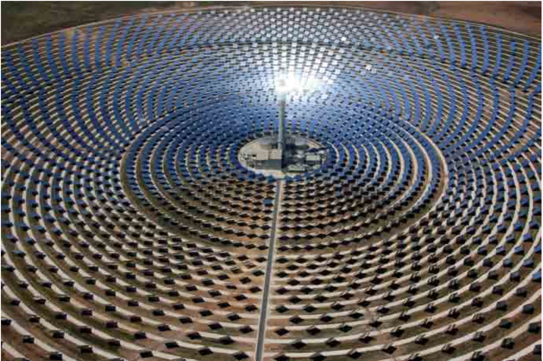
Heat storage – hot salt
